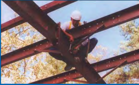
9. Install Flange Bracing
