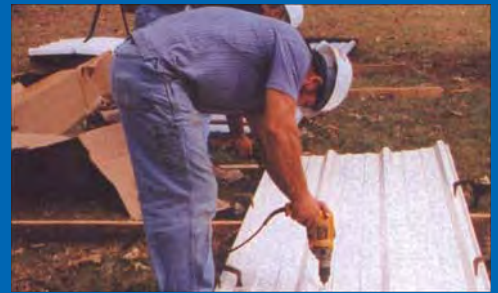
17. Pre-Drill Roof Panels
