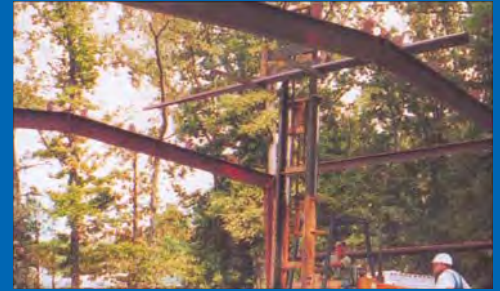
8. Install Roof Purlins
