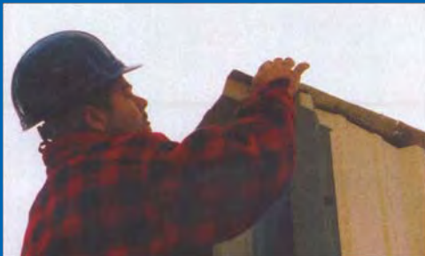
21. Install Corner Trim
