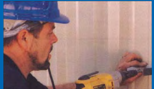
23. Attach Downspouts Straps To Wall
