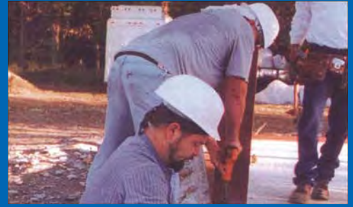
11. Install Concrete Anchors
