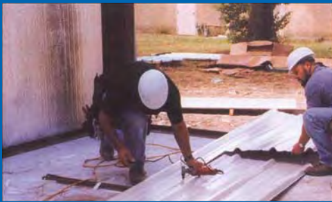
15. Cut Door Opening
