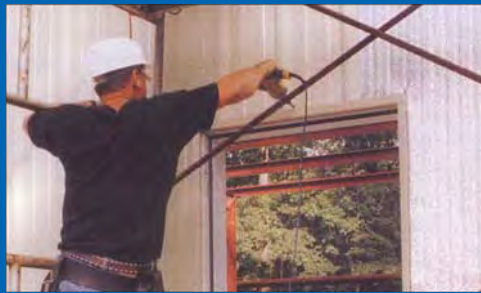
16. Install Wall Panel
