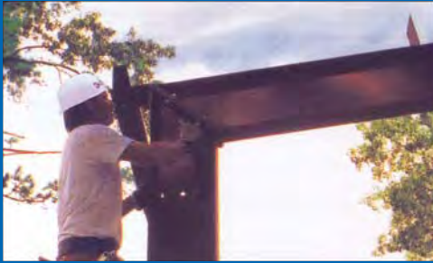
6. Connect Frame At Haunch
