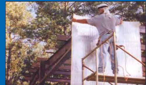
14. Install Insulation
